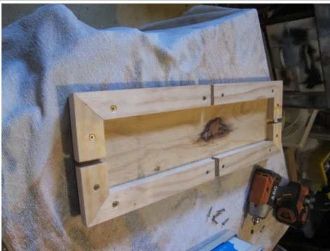
17. These timbers are now screwed in position
