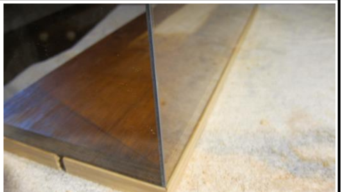
18. The case in position. Hopefully the ledge should not protrude past the case sides by more than 1mm. If the timber protrudes too far beyond the case, it can be planed back. If the timber does not protrude enough, it can be packed out with thin planking.
